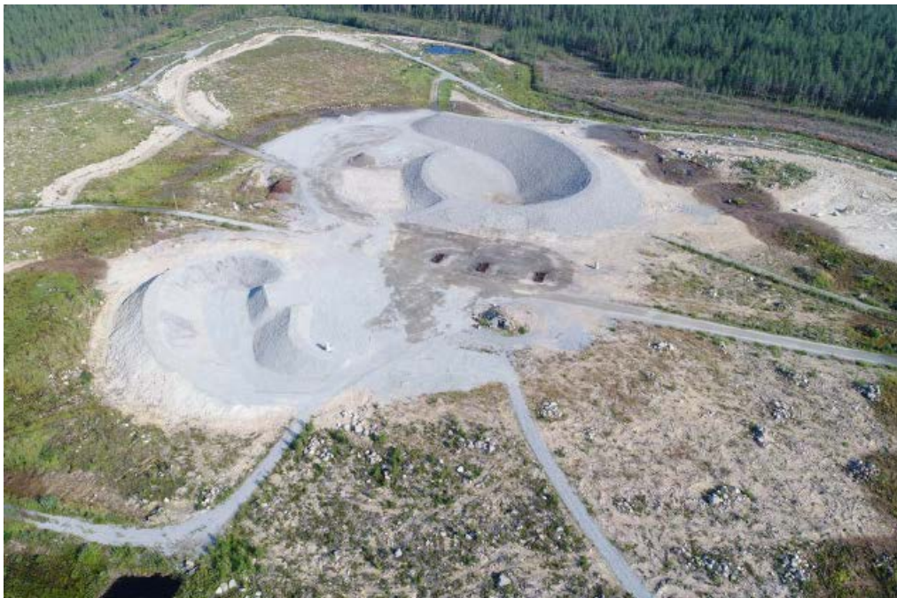
Figure 5: An example of a safety berm at a demolition area that has also noise screening properties (EPHW, 2019).
